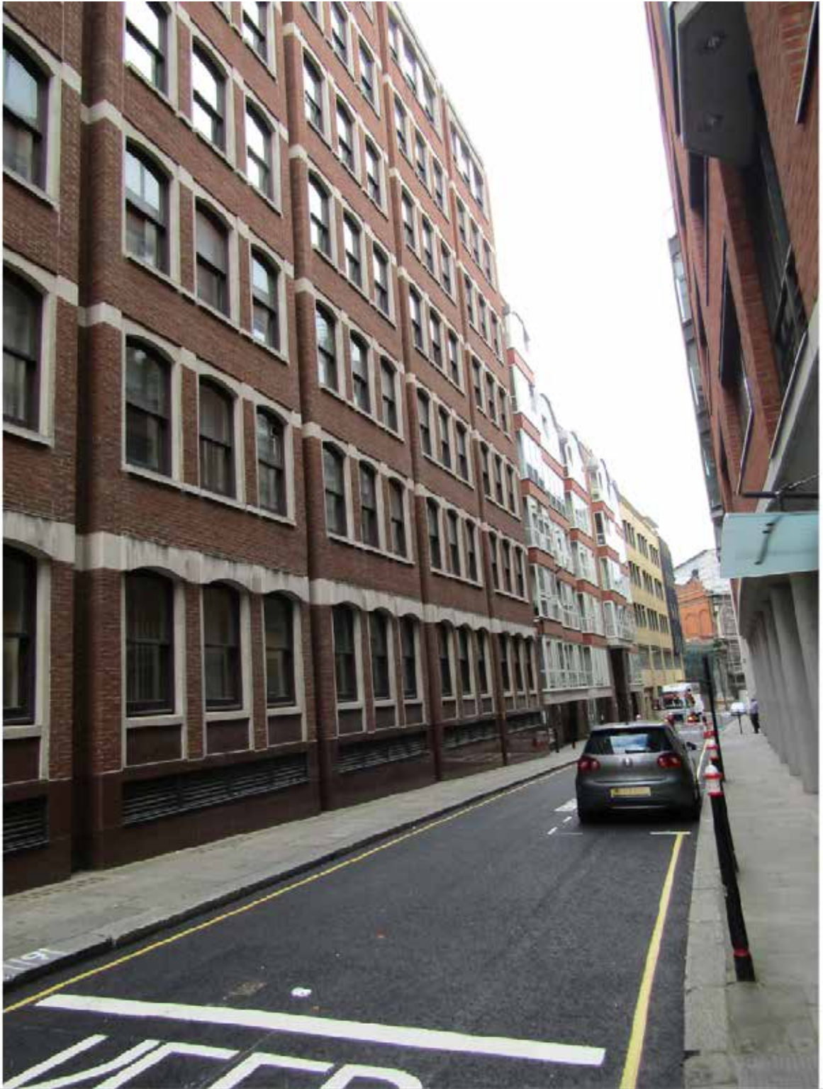
CASE No. 16/00215/FULMAJ Hosier lane, facing west
